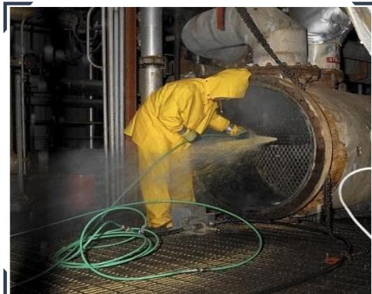
After cooling and opening all manholes, mudholes, and handholes, the vessel should be cleaned by flushing with treated water to free it from dirt, **loose scale**, debris, and other foreign material.
